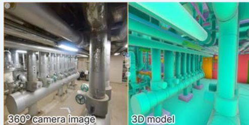
Real-time progress management using 3D digital twins
