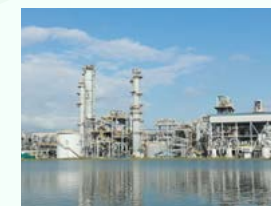
A urea plant in Bolivia (Photo courtesy of YPFB)
