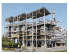
Client:S-OIL Corporation Type:Vacuum Residue Hydrodesulfurization Plant 57,000 BPSD Location: Ulsan, Korea
