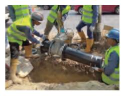
c Lient: Yangon City Development Committee Operations: Reduction of non-revenue water rate through leak survey and repair, replacement of aged water pipes and replacement and installation of meters Location: Mayangone, Yangon, Myanmar
