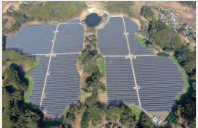
Katsuura Ueno Mega Solar Power Plant (Chiba Prefecture)
