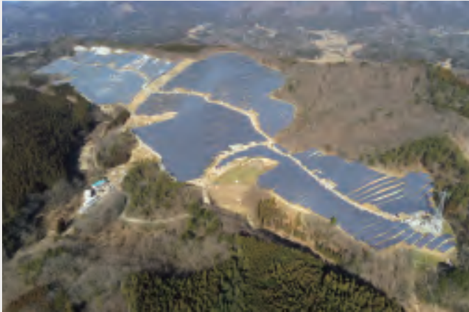
Iwaki Mega Solar Power Plant (Fukushima Prefecture)
