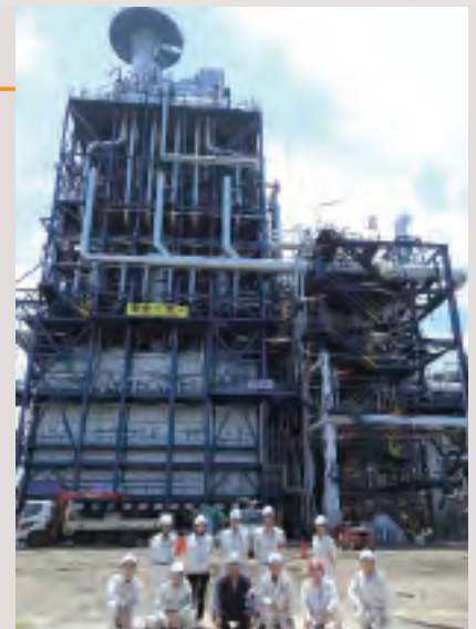
Completed naphtha cracking furnace and project team members
