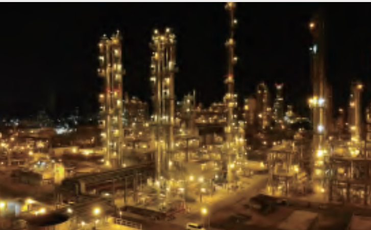
Panorama of the butene-1/MTBE plant
