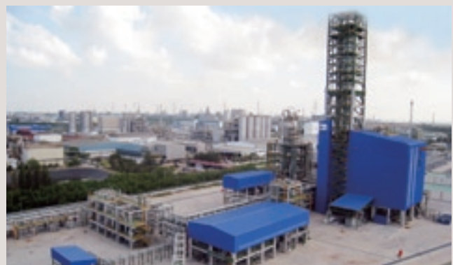
Completed LLDPE plant
