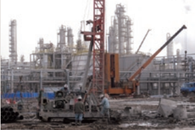
IPS-II project construction site
