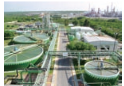
Industrial water treatment plant built for the Petróleos Mexicanos (PEMEX).
