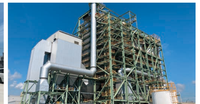
Photos of the Obayashi Kamisu biomass power plant
