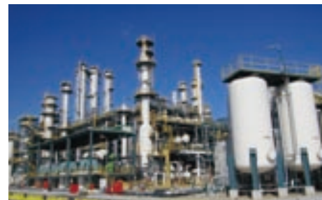
Completed refinery plant (Japan)
