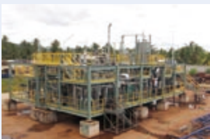
Module of Micro-GTL demonstration plant being assembled in Thailand
