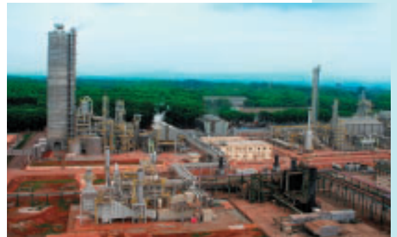
Ammonia / urea plant for PT Pupuk Kujang in Indonesia
