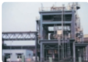
DME plant for Lutianhua Group Inc., China
