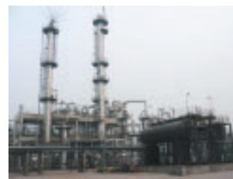
Lutianhua's 110,000t/y DME Plant
