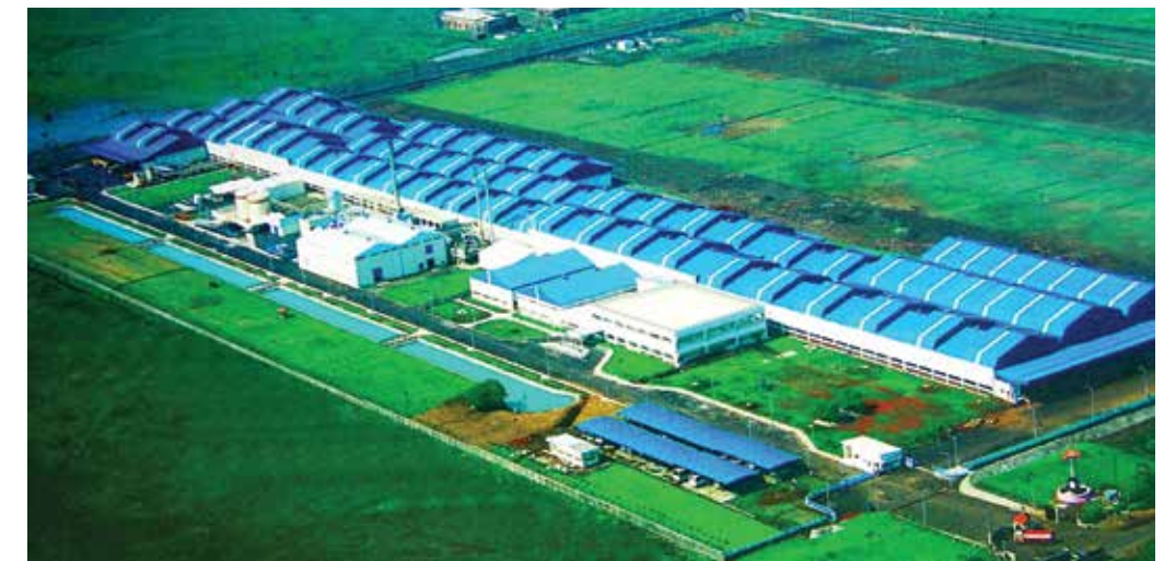
Tyre Manufacturing Plant, Kheda, Madhya Pradesh Client: Bridgestone ACC India Limited
