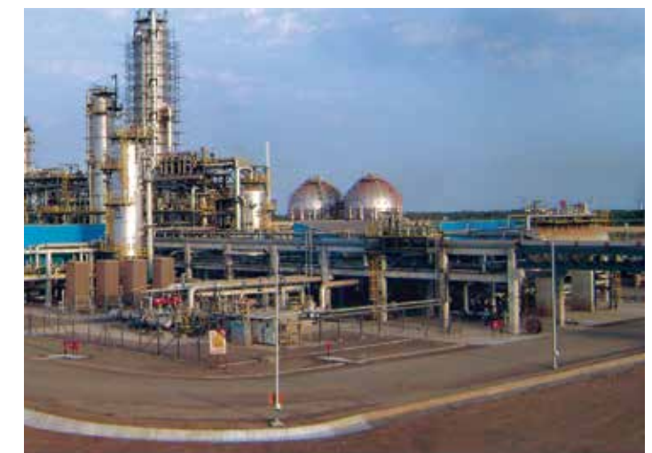
C2, C3 & C4 Extraction Plant with Truck Loading System, Dahej, Gujarat, India Client: Oil And Natural Gas Corporation
